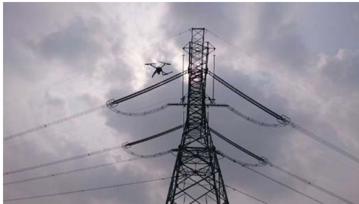
Fig. 16. Power line inspection
